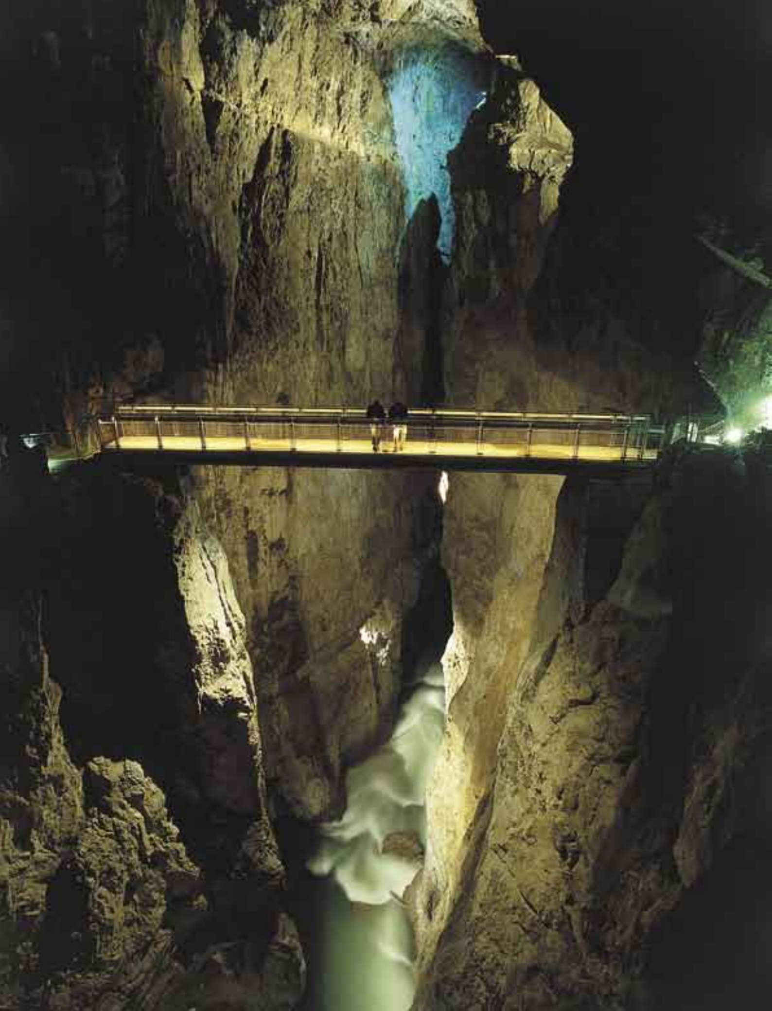
Cerkvenikov most, 45 metrov nad Reko / Cerkvenik Bridge, 45 meters above the Reka river
