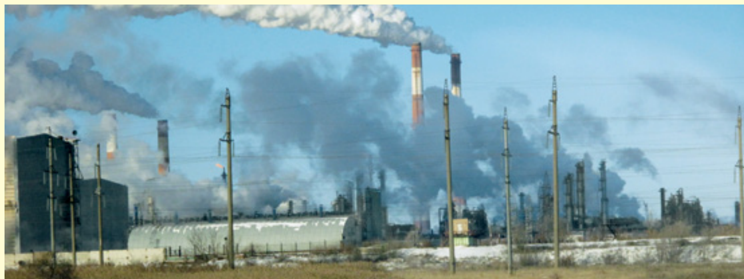
During the visit of Russian Prime Minister Vladimir Putin to Slovenia, Alexei Miller, CEO of Gazprom, and the Slovenian Geoplin company signed a joint venture to construct a gas pipeline through Slovenia.
