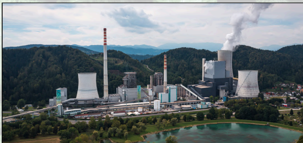
Figure 1: Šoštanj Thermal Power Plant
