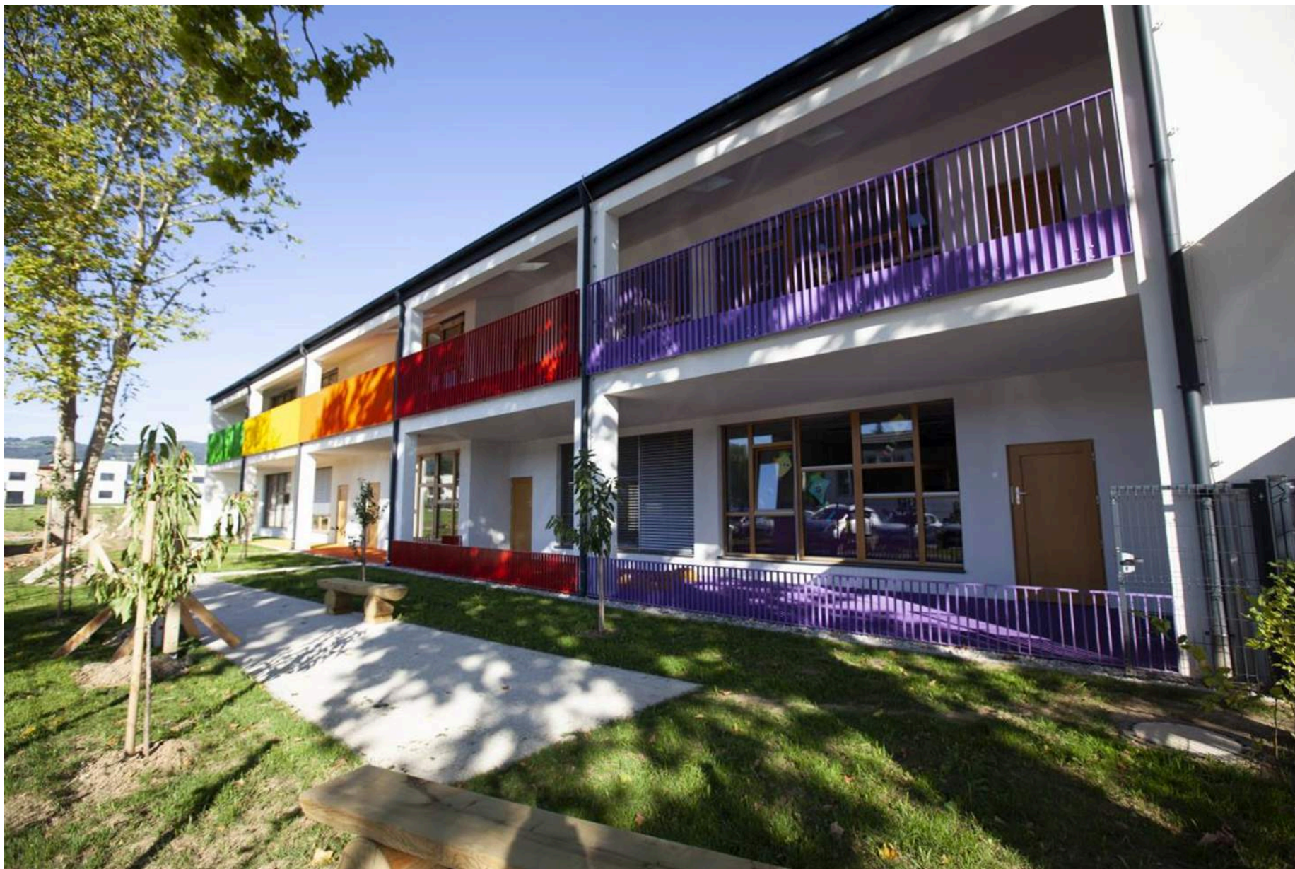
Picture 6: Kindergarten Hoče
