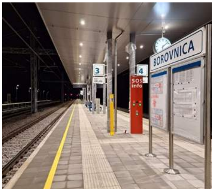
Picture 2: The railway station Borovnica
