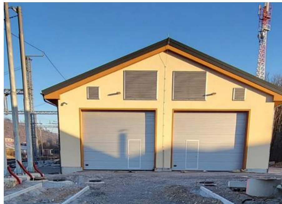
Picture 5: Power substation Postojna
