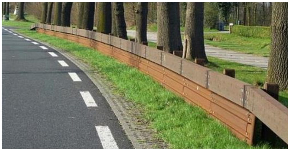
Figure 4: Proper installation of additional protection for motorcyclists on wood guard rail (source: Eurorail BV - www.eurorail.nl ).
