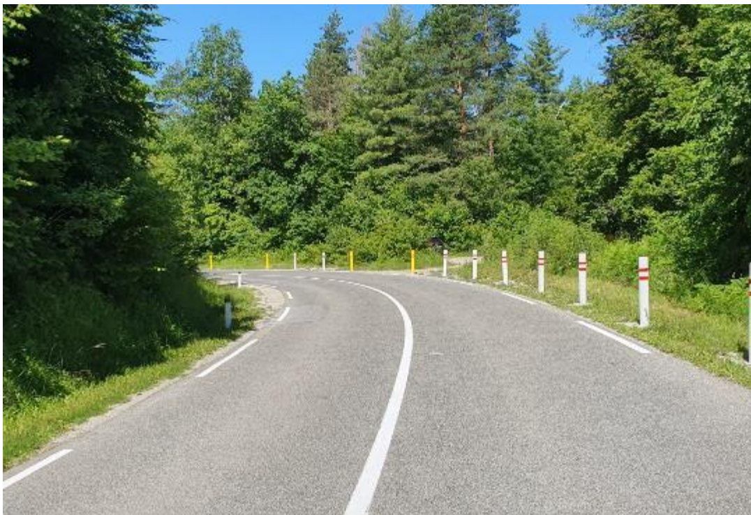
Figure 15: Passive safety poles at a junction (source: T. Tollazzi).
