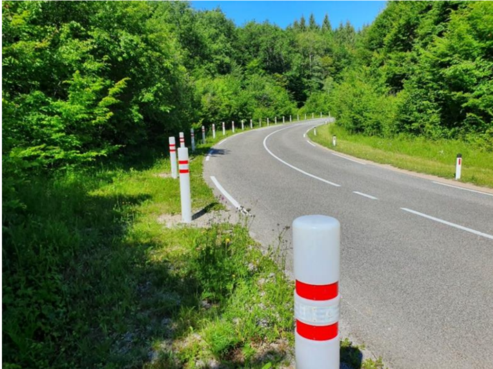
Figure 14: Passive safety poles on a curve (source: T. Tollazzi).
