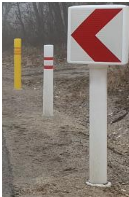
Figures 20 and 21: Distance of outer rim of PSP from edge of carriageway with additional traffic sign 3312 (source: R. Strah).
