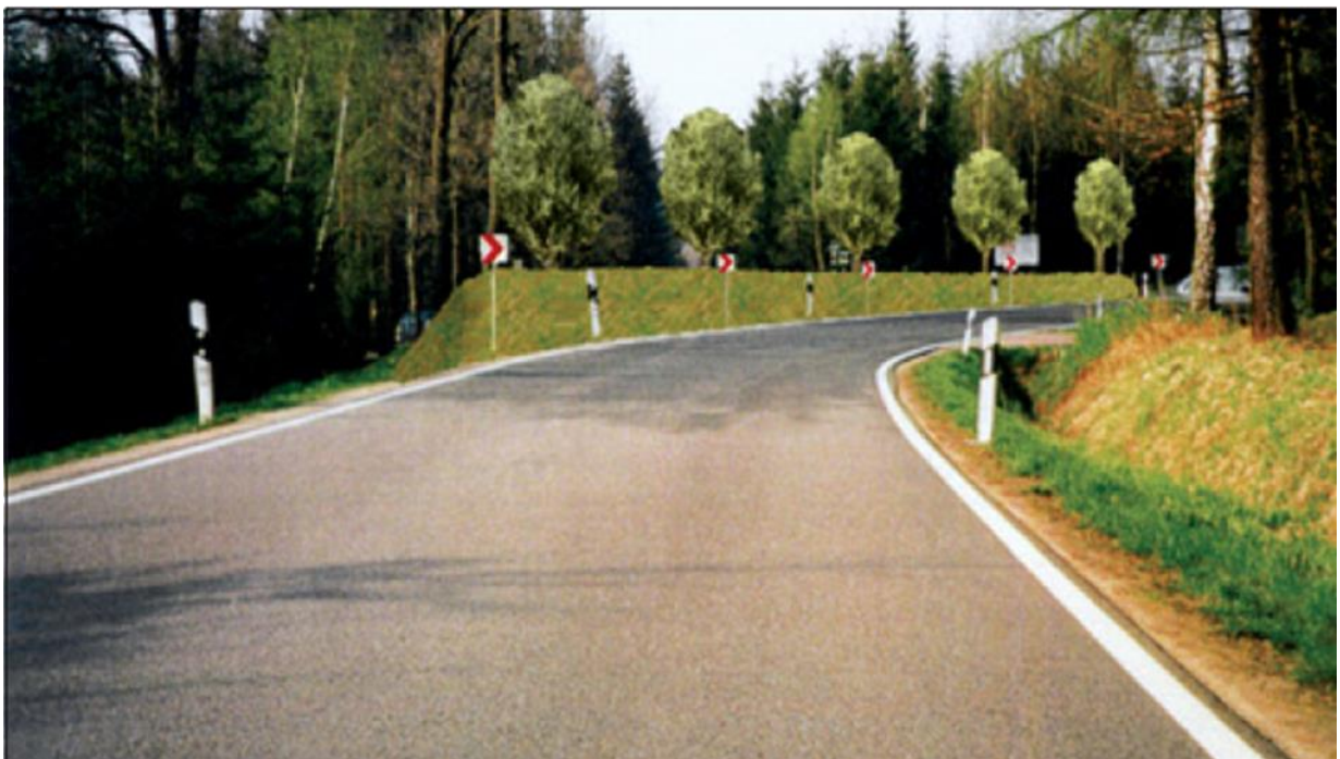
Figure 29: Execution of embankment along a curve with green cover, aimed at better guidance of motorcyclists through the curve (Source: World Road Association – PIARC: Road Safety Manual)
