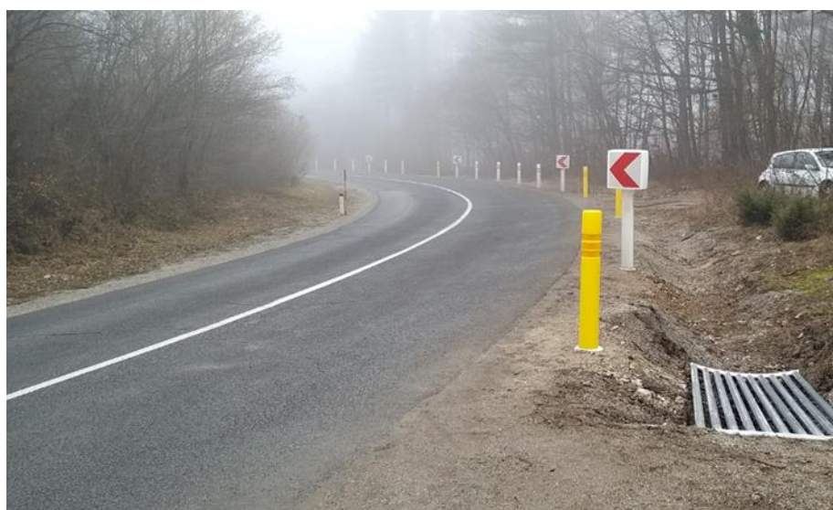
Figure 33: Example of best practice with appropriate indication of curve and junction with other safety elements for motorcyclists (source: R. Strah).
